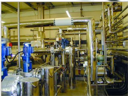
SERVICE PIPE WORK
